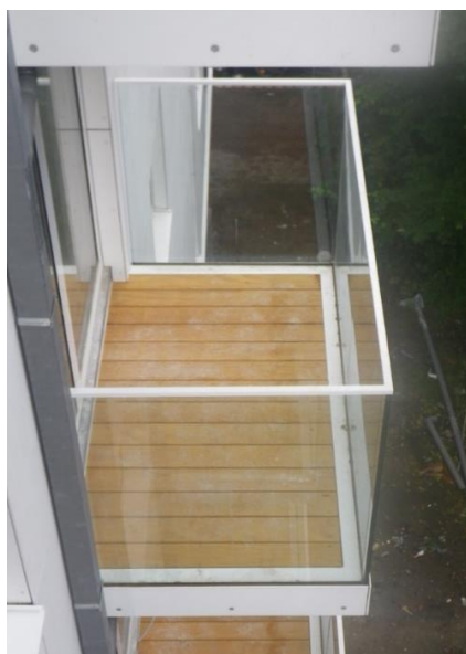
Terras - houten beplanking en glazen leuning
