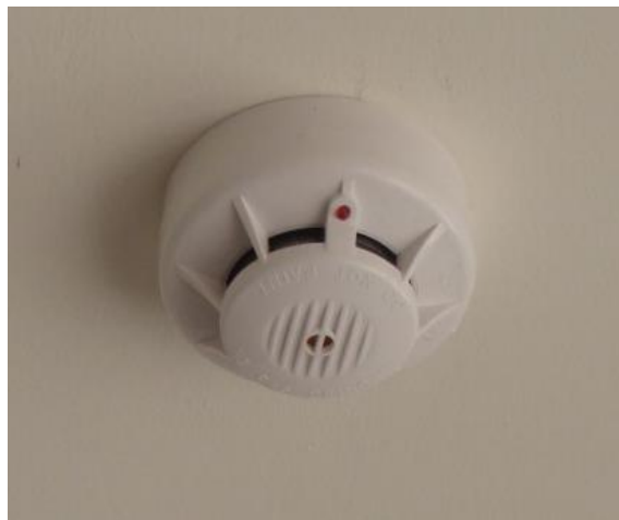
Rookmelder in appartement
